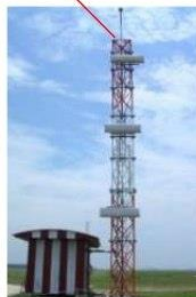
Ground Glide Path Antenna
